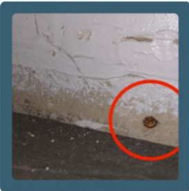
Rust & Efflorescence
