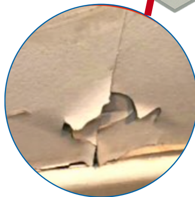
#3 Peeling & Cracking
