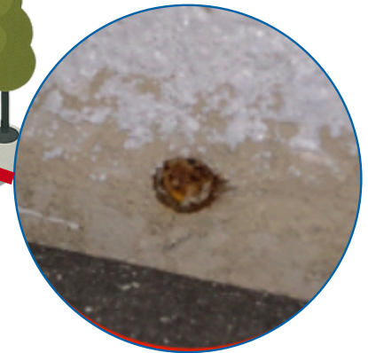
#4 Rust & Efflorescence
