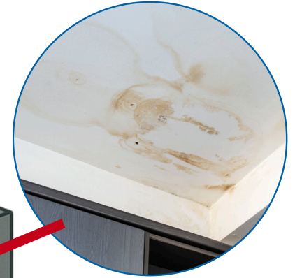
#5 Staining & Discoloration
