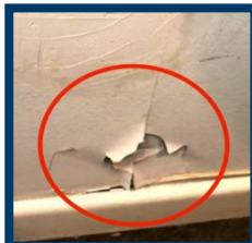
Peeling & Cracking
