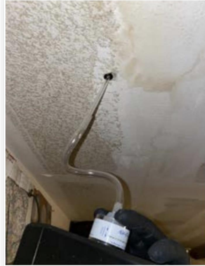
Source area of concern - Ceiling Cavity
