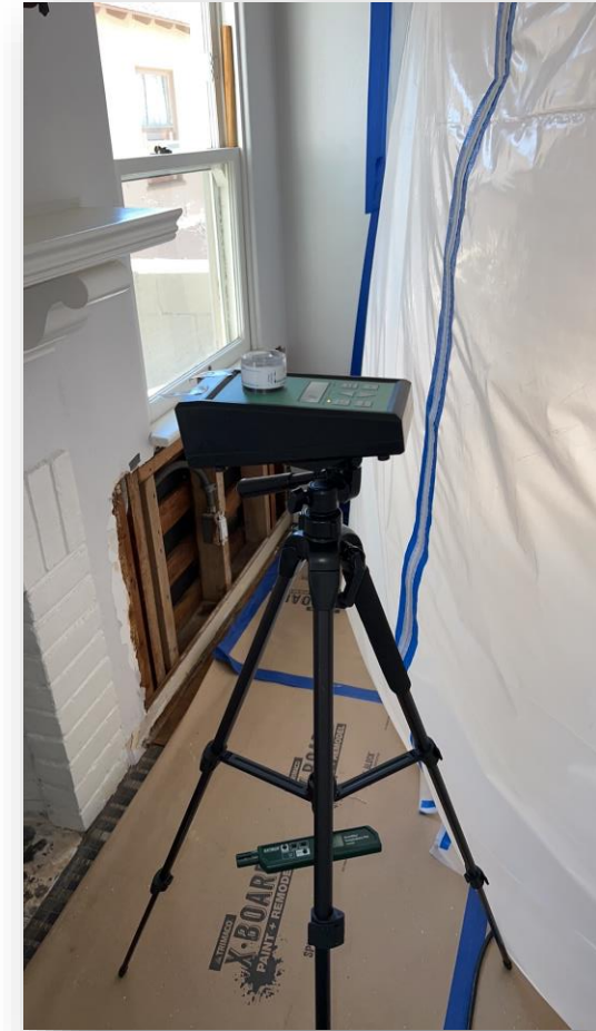
Post testing contained work areas
