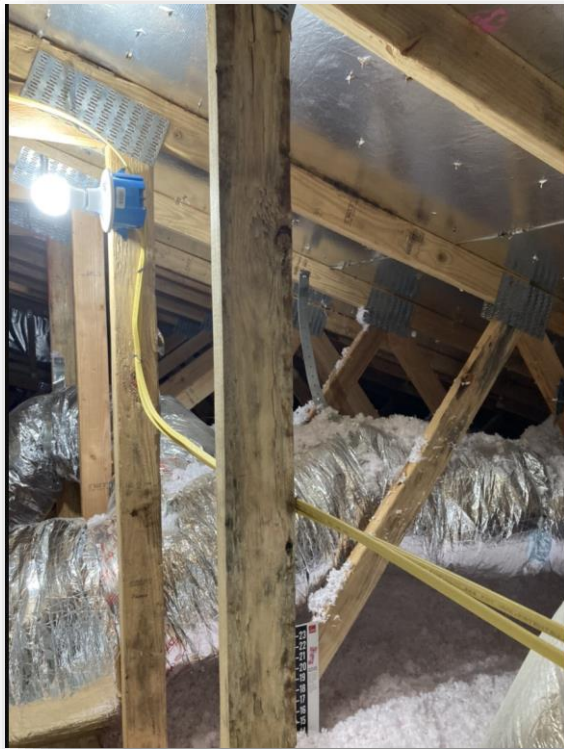
Attic Wood Frame
