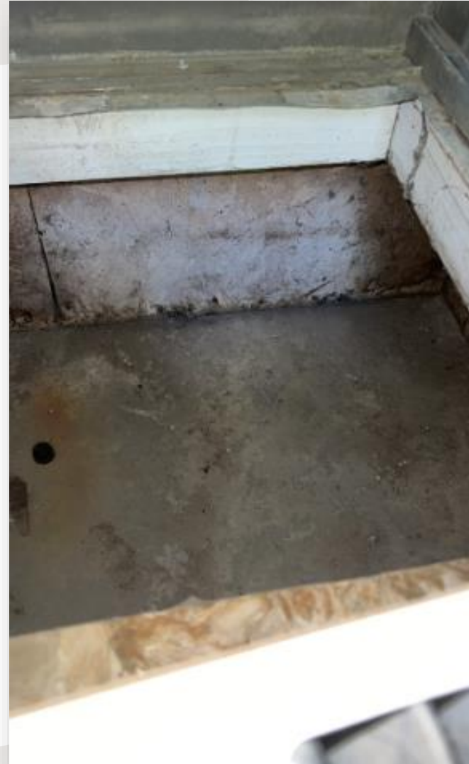
Plenum under HVAC AHU
