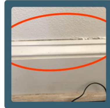
Buckling & Separating
