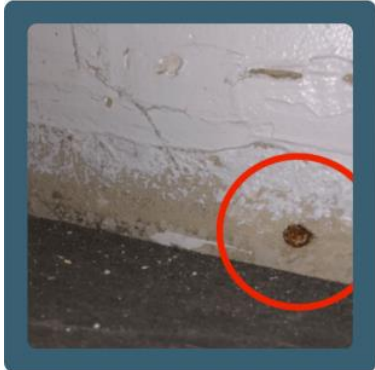
Rust & Efflorescence
